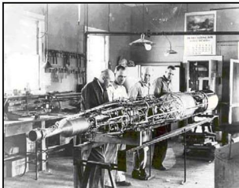
**Fig. 1. 10. Goddard examining one of his P-series rocket (turbopump fed liquid oxygen and gasoline engine) in Roswell, New Mexico, in 1940 (Courtesy NASA; <http://grin.hq.nasa.gov/UTILS/search.cgi> ).**
